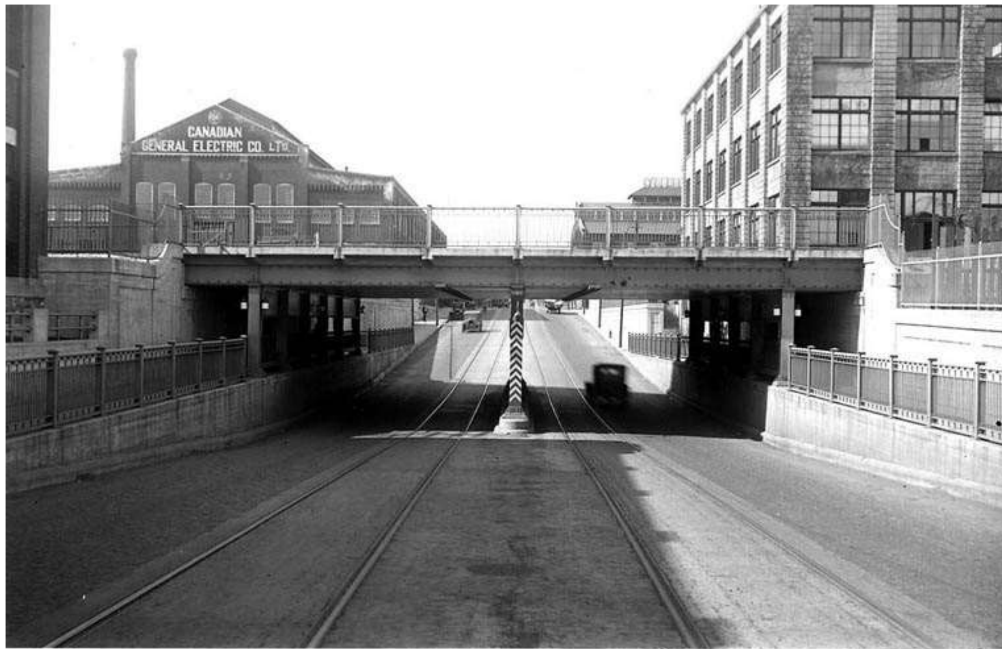
9177 Subway - Lansdowne Ave., north of Royce Ave. Apr.23/32.
